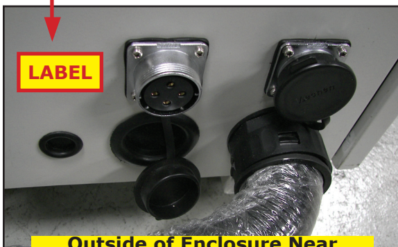
Outside of Enclosure Near Vacuum Starter Connection where the Cable comes in.
